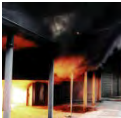
Smoke curtains are used to channel smoke away from particular areas. In this case, under a mezzanine floor.
