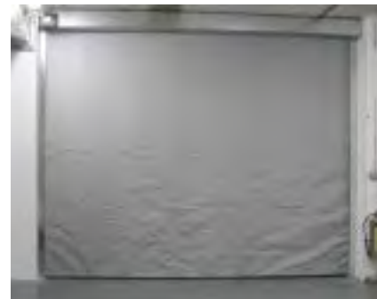
Colt Firepath fire curtains installed at Tate Gallery, London.
