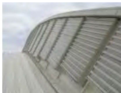
Above - Seefire natural ventilators installed into a near vertical position.
