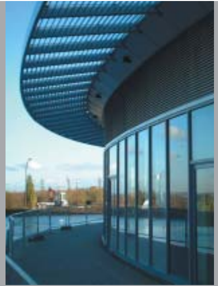
Xscape, Milton Keynes, UK Decorative Solar C Shading Louvre was installed along side Colt Universal Louvre to provide natural ventilation
