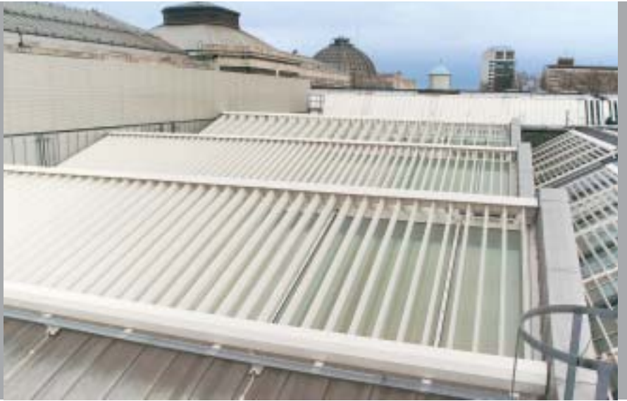
Tate Britain, London, UK. Colt controllable Solarfin hollow section aluminium fins installed on top of Colt Azur rooflight systems
