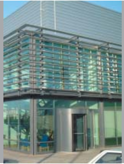
Conix, Liverpool, UK. Designed by architects Austin Smith Lord, the Conix building incorporates a fixed Solarfin system to prevent solar heat gain and glare to the front offices and to visually enhance the overall building
