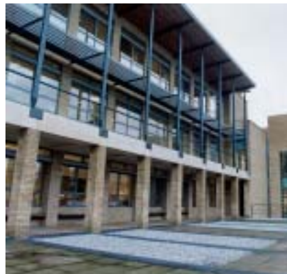
Canon Headquarters, UK. A bespoke variant of the Solar C Fixed Louvre was installed along the front façade and over the rooftop systems
