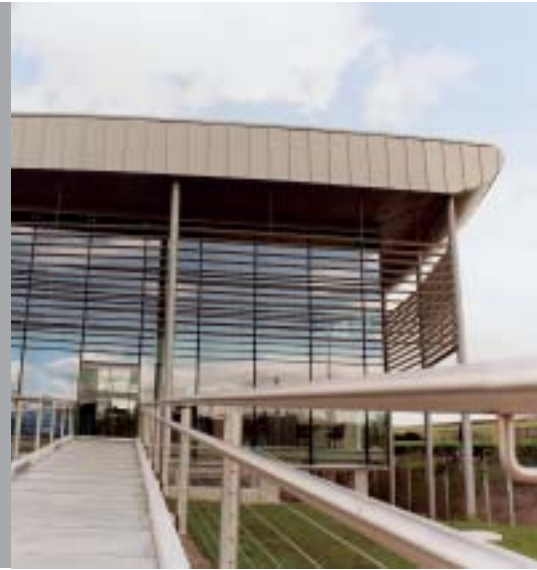
West Coast Rail Traffic Control Centre, Saltley
