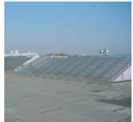
BMW Education & Production Centre, Germany. In addition to controllable Solarfin, Colt Solar C was installed over the top of a Colt Azur rooftop system to prevent solar glare.
