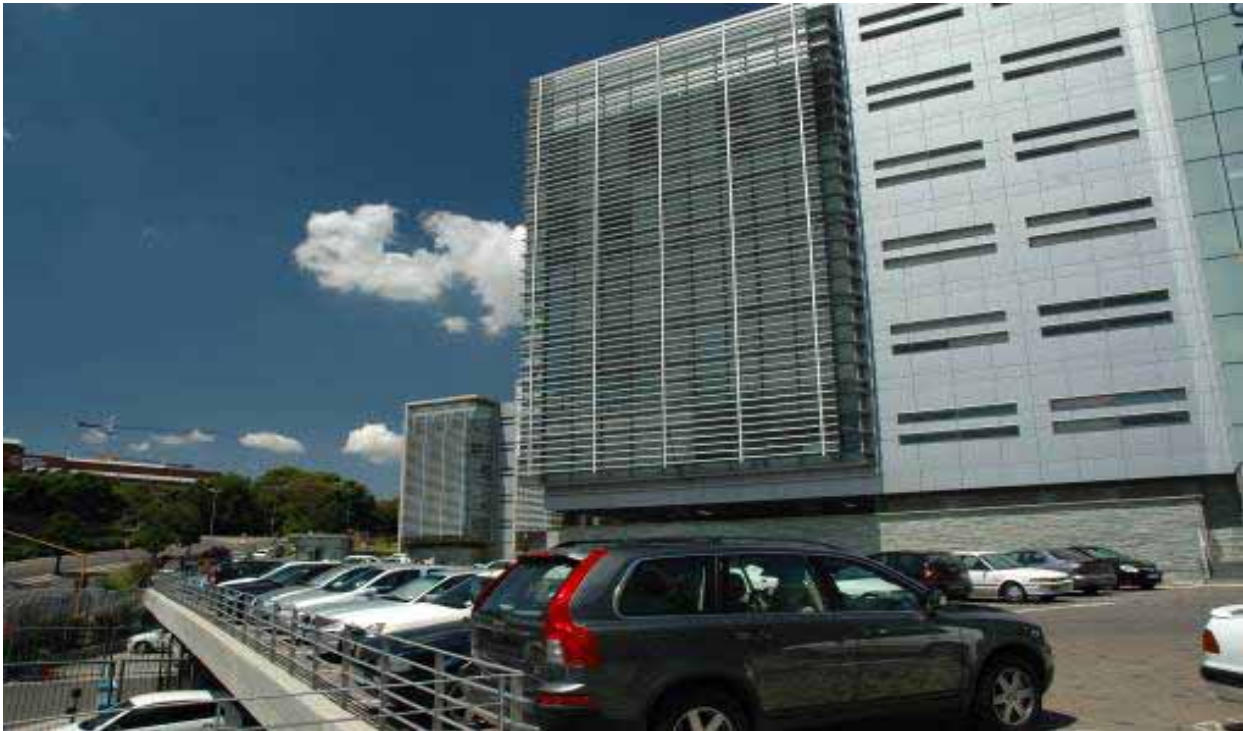
Project: Upgrade, Maintenance & Refurbishment of Existing Colt Solarfin Shading System. Location: Discovery Health Head Office, Sandton.
