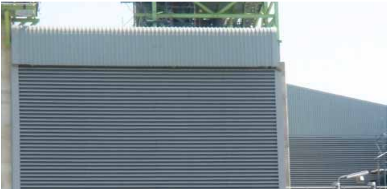
Project: Design, Supply, Delivery & Installation of 10 000m 2 of Robertson Continuous louvres Location: Mozal Aluminium smelter Mozambique
