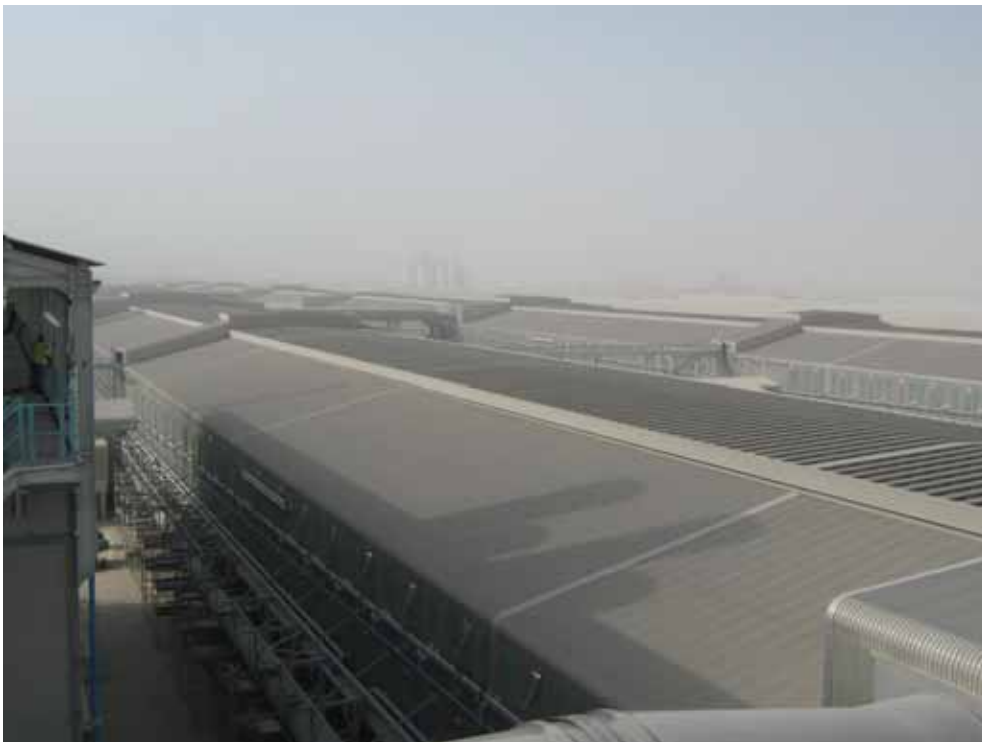
Project: Design, Supply, Delivery & Installation of 51 030 m 2 of Robertson SF 1000 Continuous Ventilator and 325 000 m 2 of A7 Wall and Roof Cladding Location: Oatalum - Qatar
