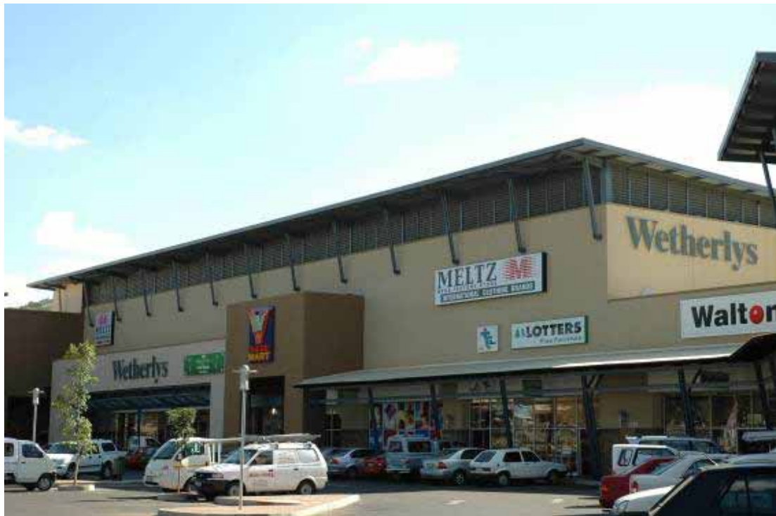
Project: Design, Supply, Delivery & Installation of Sigma Screening Louvre System. Location: Rustenburg.
