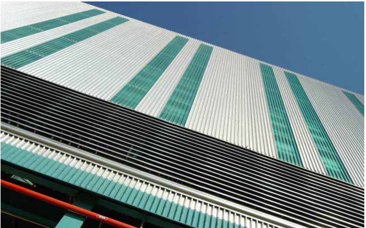
Project: Design, Supply, Delivery & Installation of 10 000m 2 of Robertson Continuous louvres Location: Mozal Aluminium smelter Mozambique
