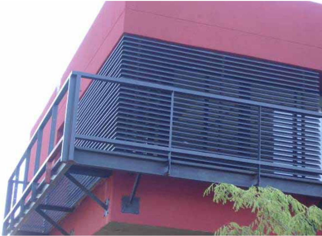
Project: Design, Supply, Delivery & Installation of Solar C Shading System. Location: Private Residence, Mooikloof
