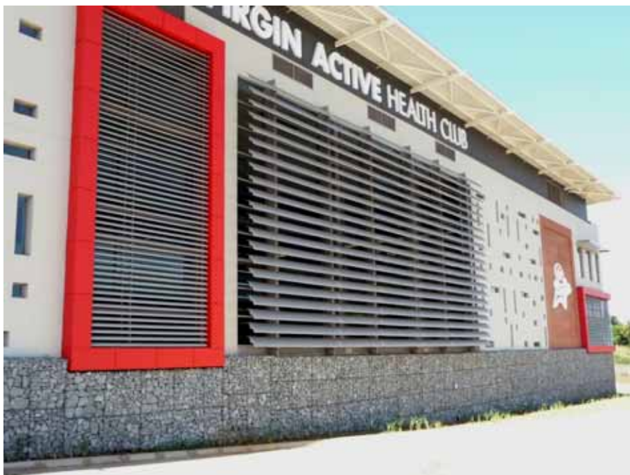
Project: Design, Supply, Delivery & Installation of Multiple Fixed Systems of Solar C130 and C100 Screens and CPL 400/80 Perforated (Centre) Screen
