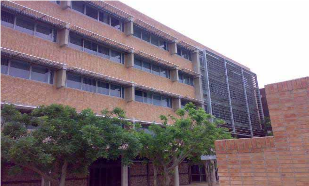
Project: Upgrade, Maintenance & Refurbishment of Existing Automated Colt Solarfin & Solar C Shading System - Location: Bafokeng Municipality Head Office.
